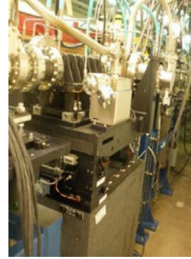
Figure 1: Installed GRID-XBPM at 27-ID FE (Looking upstream) [2].
