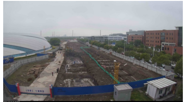
Figure 9: SXFEL construction site at 9:00 A.M. on May 28, 2015.
