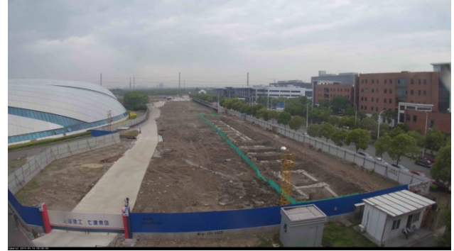
Figure 8: SXFEL construction site at 9:00 A.M. on May 14, 2015.
