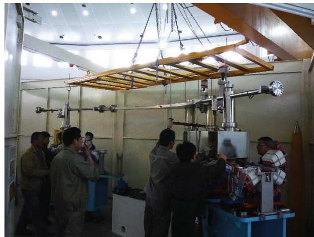
Figure 5: Installing of a subsystem.
