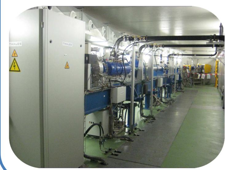
The LINAC cooling water system has two different functions. From one side it cools the elements with strong dissipation of power: klystrons, RF cavities, RF loads, RF ceramic windows and magnets. And from the other side the system regulates the water temperature of the RF cavities in order to tune them for working at the nominal RF frequency.
