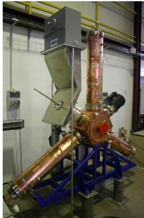
6x Main NC RF cavity 400 kV - 500 MHz
