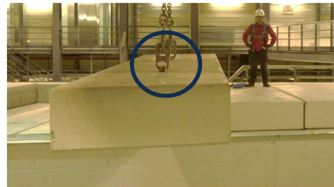
Tunnel Roof Lifting with Mechanical bolts
