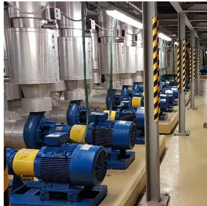
Cooling Production Water Pumps 7°C
