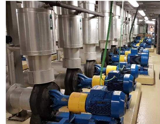
HVAC and Cooling Water Pumps 7°C
