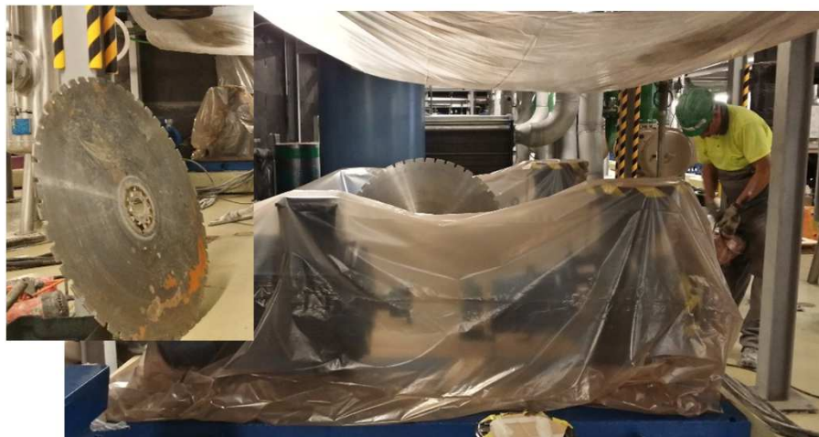
Cutting the concrete
