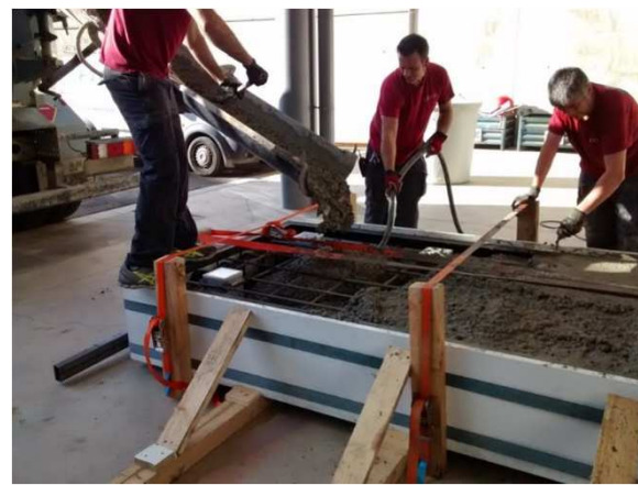
Concrete Filling
