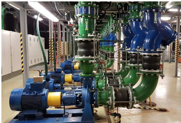
Cooling Tower Water Pumps 25°C
